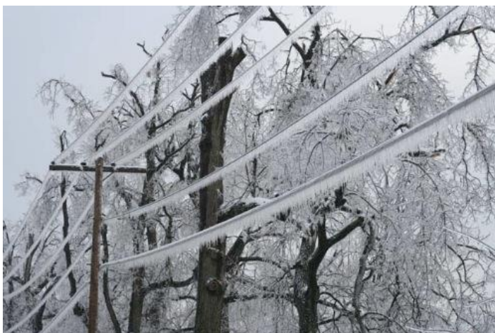
Figure 3-19 Ice Covered Power Lines
