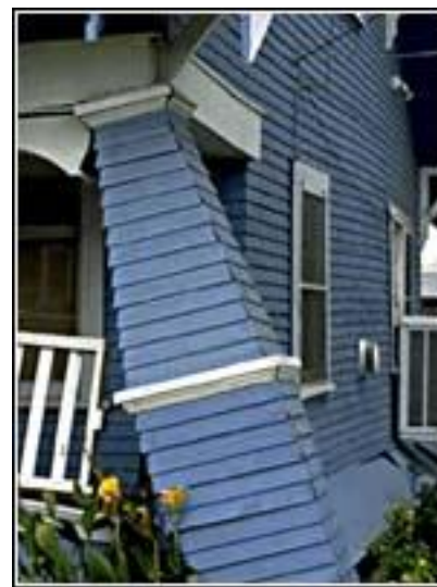
Figure 3-6 Earthquake Damaged Porch
